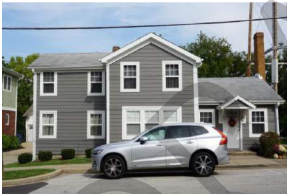
FIGURE 52: Example of the Central Block with Wings type in the survey area at 127 Kansas Street. The original typology has been altered by the addition of a second floor at the west (left) wing.
