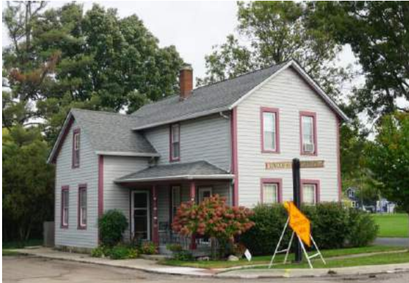
FIGURE 53: Example of the Three-Bay type in the survey area at 21 Carpenter Street. The form of the typology has been altered due to the construction of a front addition at the north end of the front (west) façade, visible in the photo.
