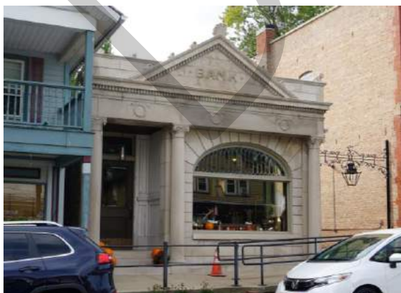
FIGURE 67: Example of the One-Part Commercial Block type in the survey area at 114 Kansas Street.
