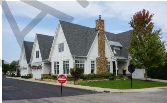
FIGURE 63: Example of a Townhouse in the survey area at 51-53 Elwood Street.
