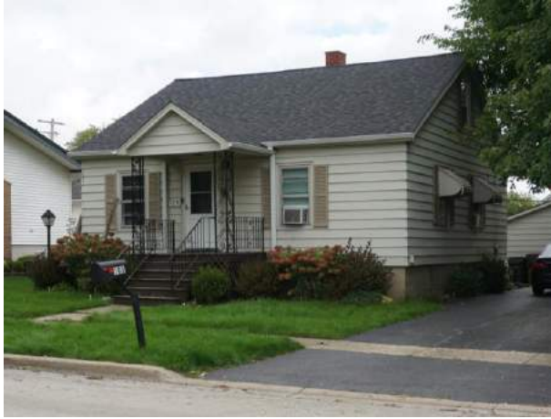
FIGURE 90: Example of the Minimal Traditional style in the survey area at 105 Hickory Street.
