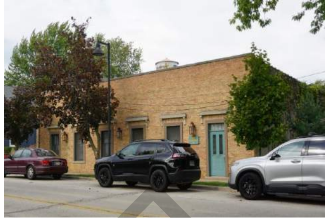
FIGURE 99: Example of the Utilitarian style applied to a non-residential building, the former Frankfort Fire Protection District, in the survey area at 106 Kansas Street.
