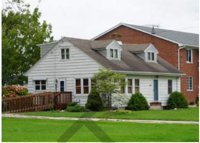
FIGURE 91: Example of the Cape Cod subtype of the Minimal Traditional style in the survey area at 240 N. White Street.
