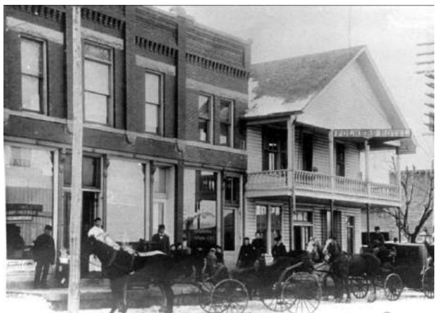
FIGURE 25: Photograph of the Folkers Meat Market (left) and Folkers Hotel (right), located at 116-118 and 122 Kansas Street, respectively. Source: Frankfort Area Historical Society.
